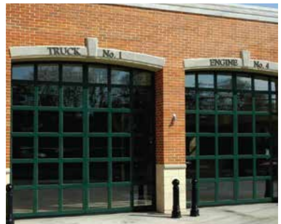
Edison Fire Department, NJ Photo and installation by Advanced Door Sales
