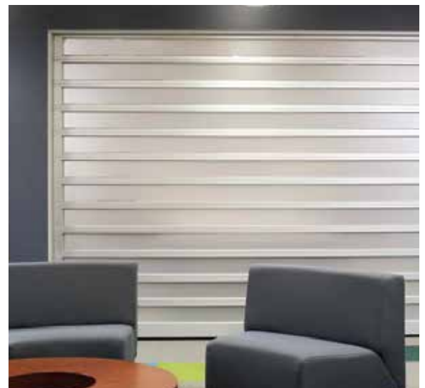
Photo and installation by Door Systems of Itasca
