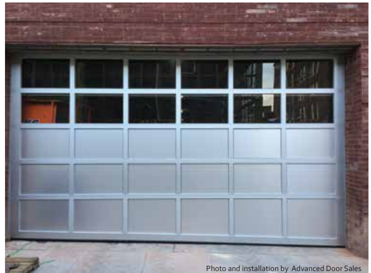
Photo and installation by Advanced Door Sales
